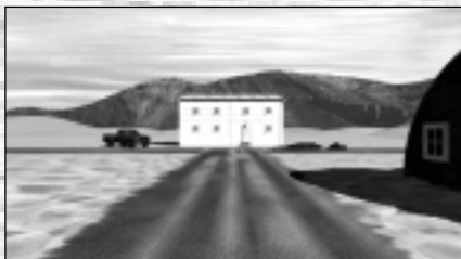
Warehouse (outside view)
