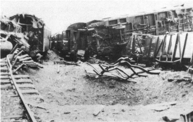
A rail yard at Buir, near Cologne, destroyed by U.S. bombs. Note the bomb crater in the foreground.
